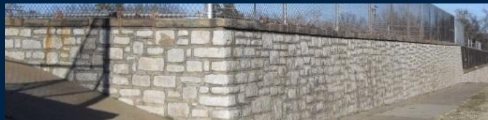
Keep all WPA walls & stairs
